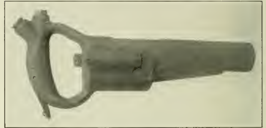
An Improved Air Hammer for Riveting.
